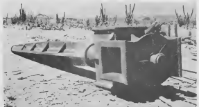
WHEN THIS 10,000-pound iron shaft was hand-forged in 1815 it represented quite a feat of technical skill using the crude tools available. TEMPO CU e shaft di hero aki di 10,000 liber a worde forja na 1815 tabata un aconpliecimento grandi usando e hermentnan crudo.
